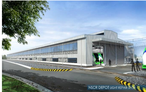
NSCR DEPOT LIGHT REPAIR SHOP
