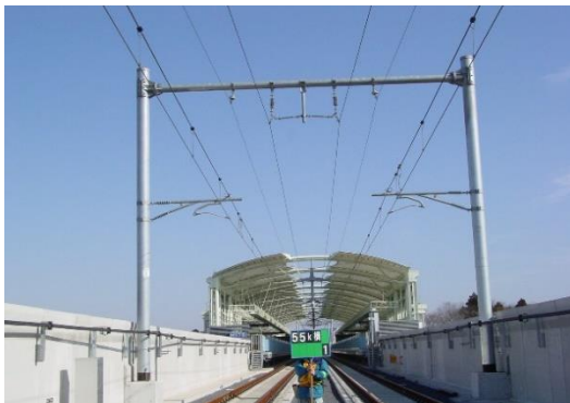
Steel Tube Mast
