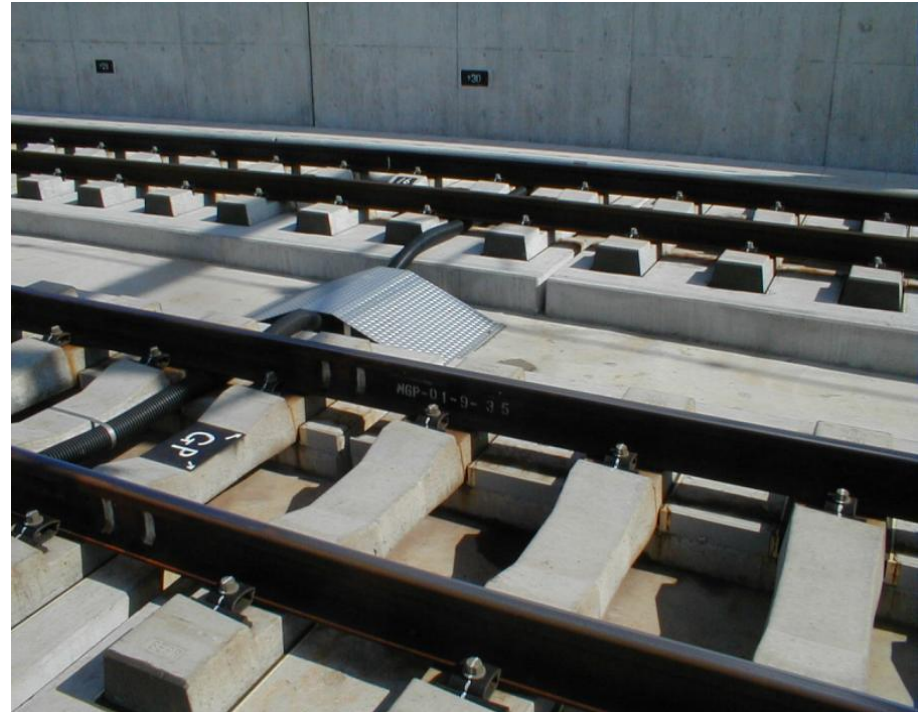
SLAB TRACK AT STATION
