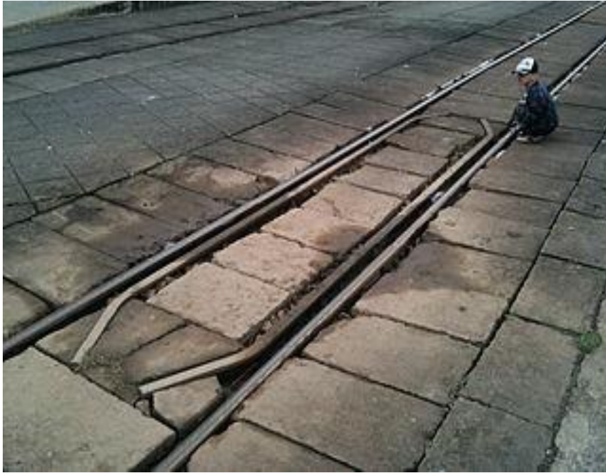
Check Rail @ Level Crossing
